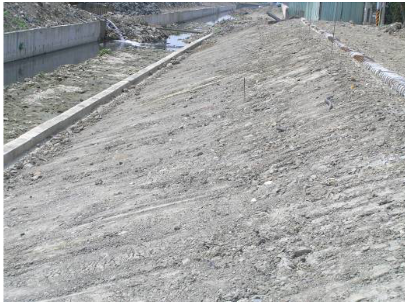
Picture 1. Site preparation
