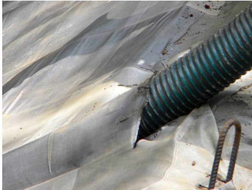
Picture 5. Inserting filling pipe
