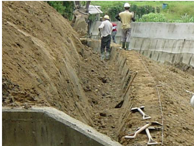
Picture 2. Excavation of the anchor trench at the top of slope
