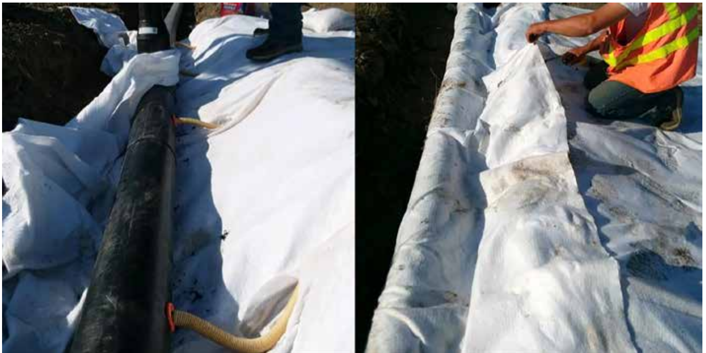
Figure 13: Connection to a plain drain with Quick Connect
