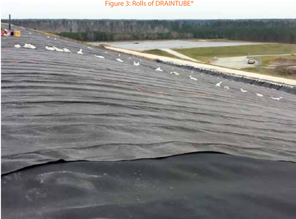
Figure 4: DRAINTUBE® unrolled
