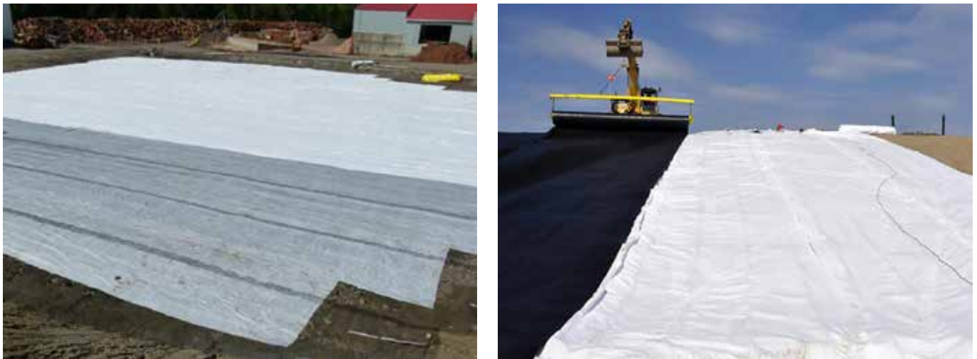
Figure 14: Upper geosynthetic layer placement
