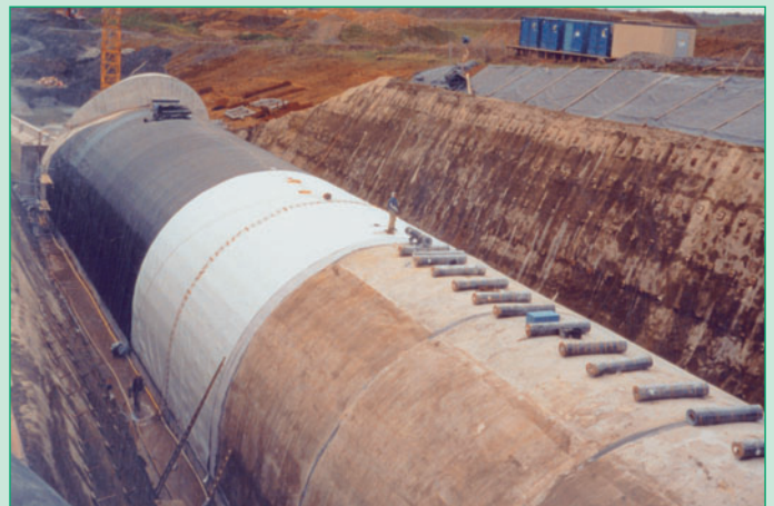
Fig. 23: Portal area with Carbofol® tunnel geomembrane
