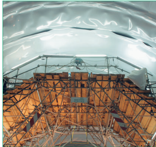
Fig. 31: Carbofol® tunnel geomembranes over an arch scaffold
