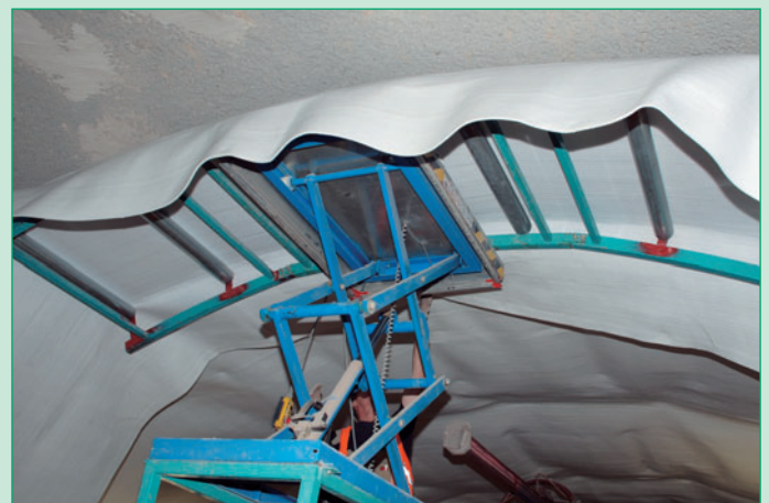
Fig. 26: Securing the Secutex® protection geotextile (arch area)
