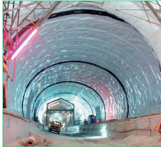
Fig. 2: Arch sealing, using Carbofol® tunnel geomembrane
