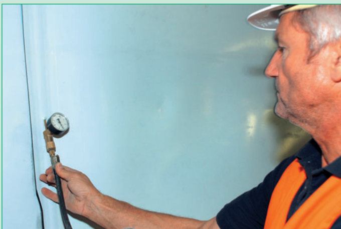
Fig. 33: Air pressure testing of a double wedge weld seam
