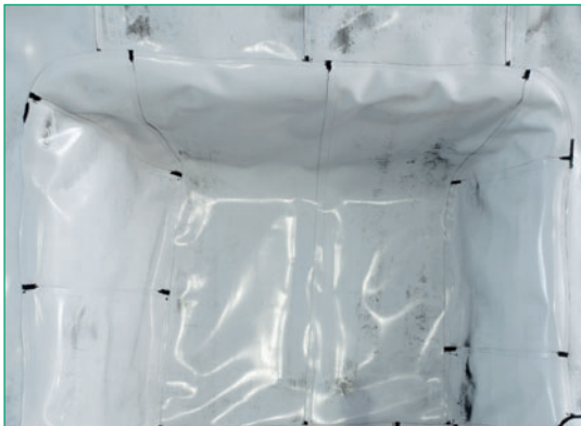
Fig. 32: Carbofol® tunnel geomembranes in the niche area
