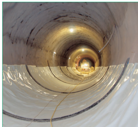
Fig. 3: Carbofol® tunnel geomembrane in the floor area
