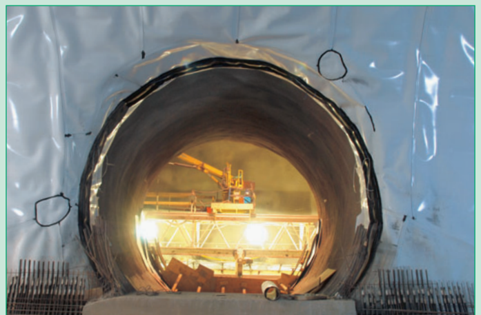
Fig. 21: 360° sealing in a connection tube
