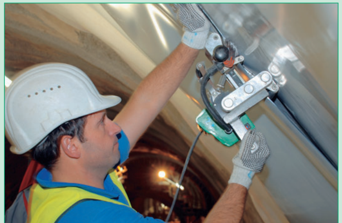
Fig. 30: Welding of Carbofol® tunnel geomembrane using a hot-wedge welding machine
