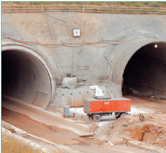
Fig. 1: Tunnel portal area
