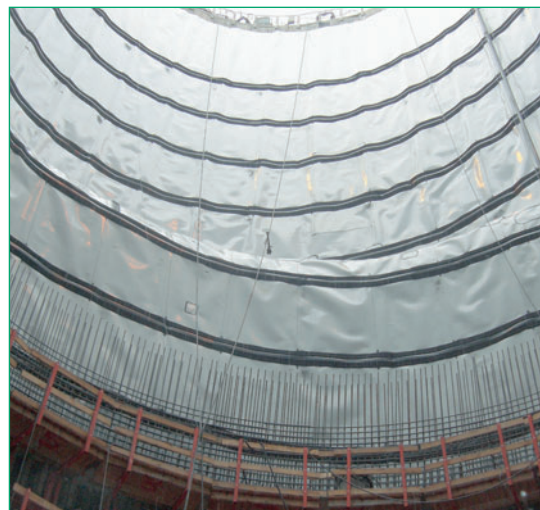
Fig. 35: Waterstop system in the shaft area
