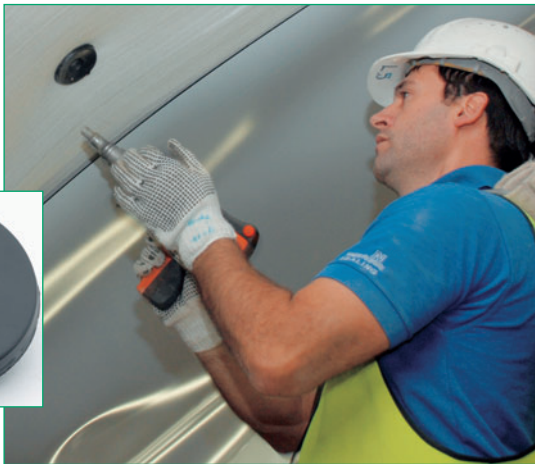
Fig. 27: Attaching the protection geotextiles using Carbofol® rondelles and a bolt gun
