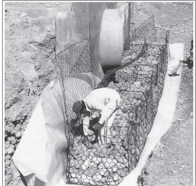
a) Hand positioning of rock against face of Gabion cages
