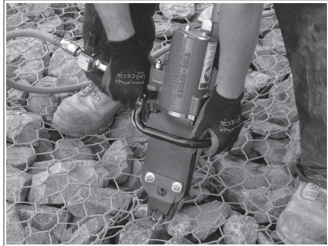
Figure 41 - Pneumatic closing tool for installing "C" ring connectors.
